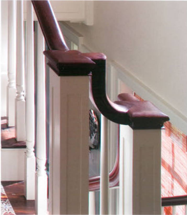
Stair newel and handrail
