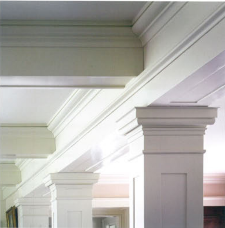
Living room column detail
